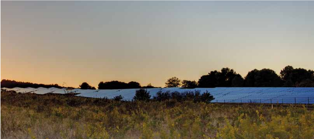
The Solar Power Plant with the 29,931 modules is the first Free-Field Solar Power Plant, based on Solar Frontier's CIS technology. (Image: BELECTRIC France)
